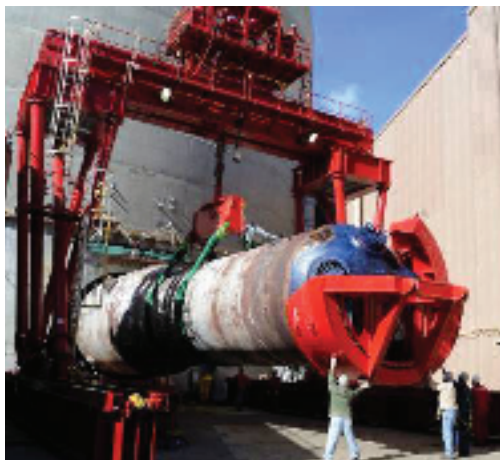
DCPP's award winning steam generator replacement project in 2009.
